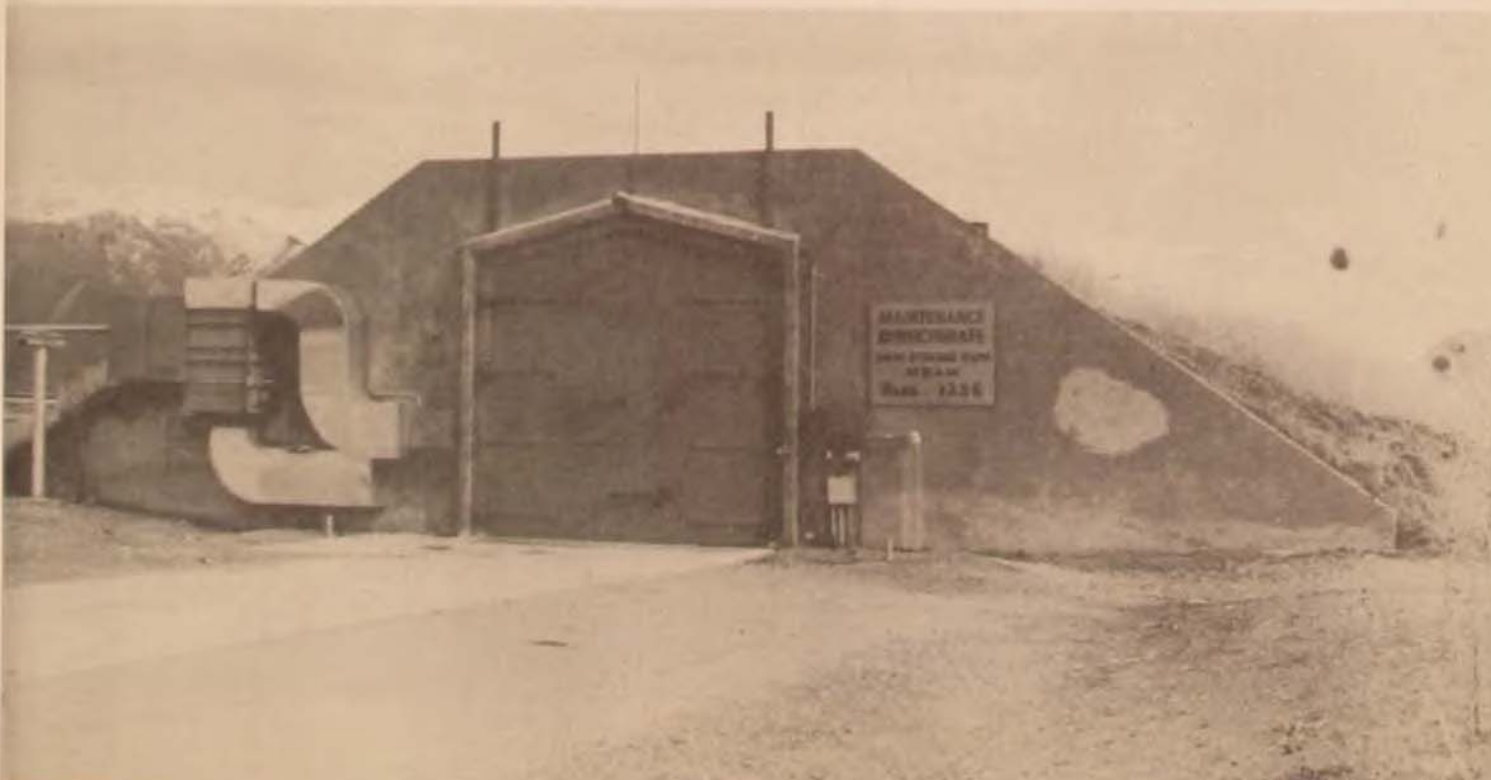
An igloo at Ogden Air Materiel Area, Hill AFB, Utah, for storing LGM-30 Minuteman missiles, engines, and other hazardous missile components.
